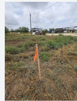
Figure 10 Survey Stake Marked 18 04+010
