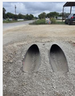
Centro Esperanza Recently Installed Driveway Storm Drain Right Side
