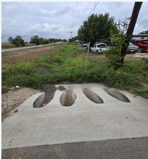
Figure 3. Left Side Storm Drain
