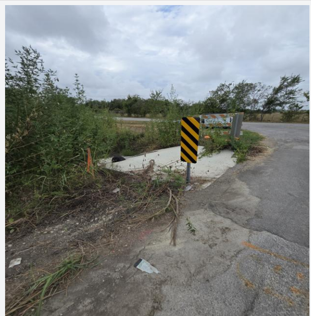
Figure 2. Right Side Storm Drain Path Recently Installed .
